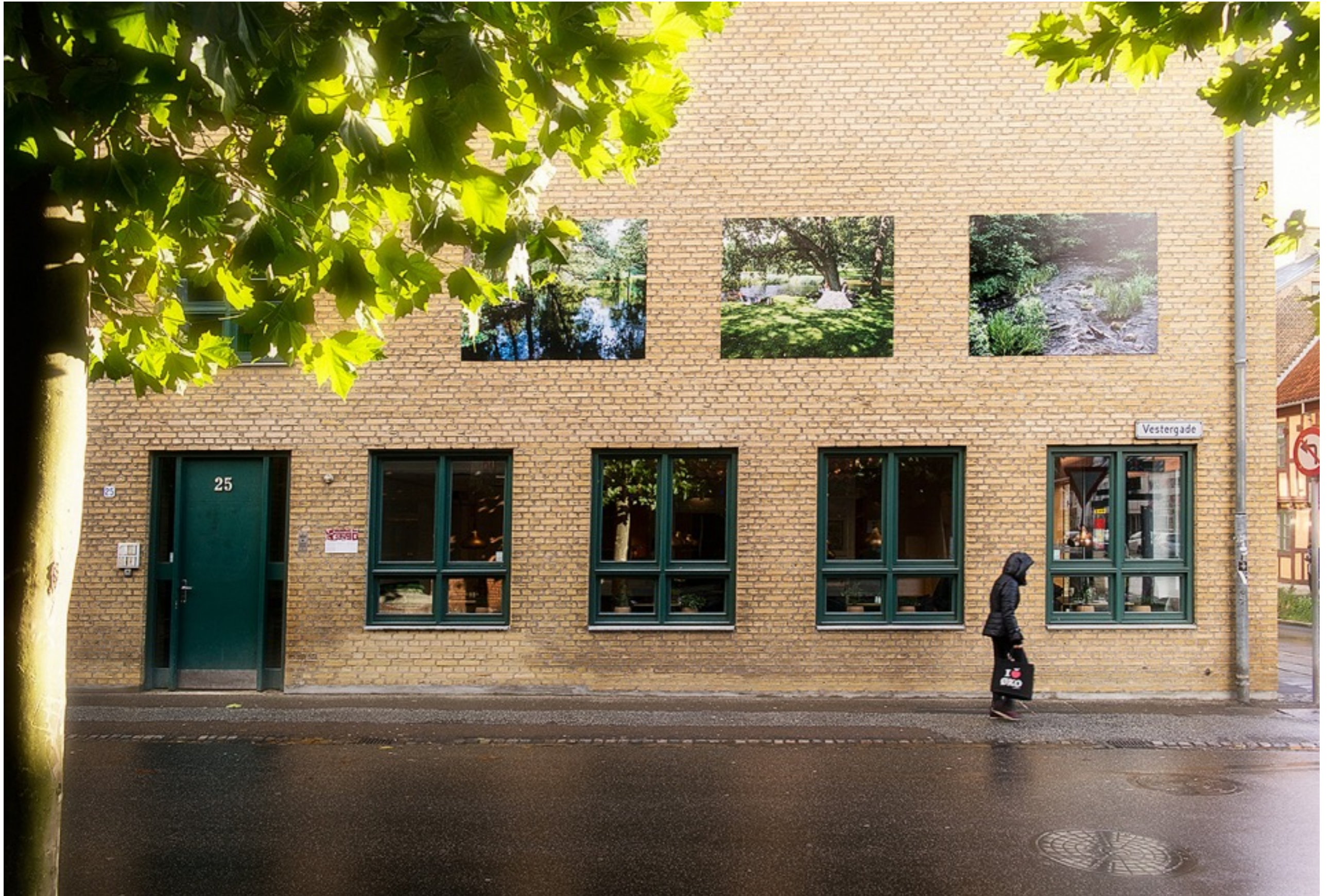
STATION 2: Works by Hyun-Jin Kwak installed on the facade of a local community centre and nursing home.
